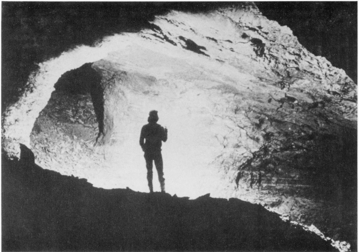
Plate 3b: Lincoln Hill Limestone Mine in 1975. A member of the Shropshire Mining Club is standing on a pile of debris facing a solid pillar of limestone; fourteen such pillars. 6–9 m high and about 6 m square, support the roof. (D. Stevenson).
