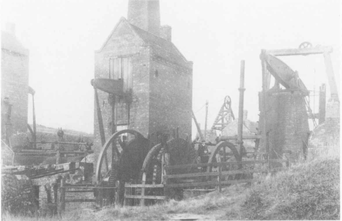
Plate 4a: Part of Madeley Court Colliery in about 1906. Coal, ironstone and fireclay were extracted from shafts 50–90m deep. In 1882 the surface equipment comprised one pumping engine, seven winding engines and one 'old water engine', all steam powered and of the beam type. (The late W. Harper).
