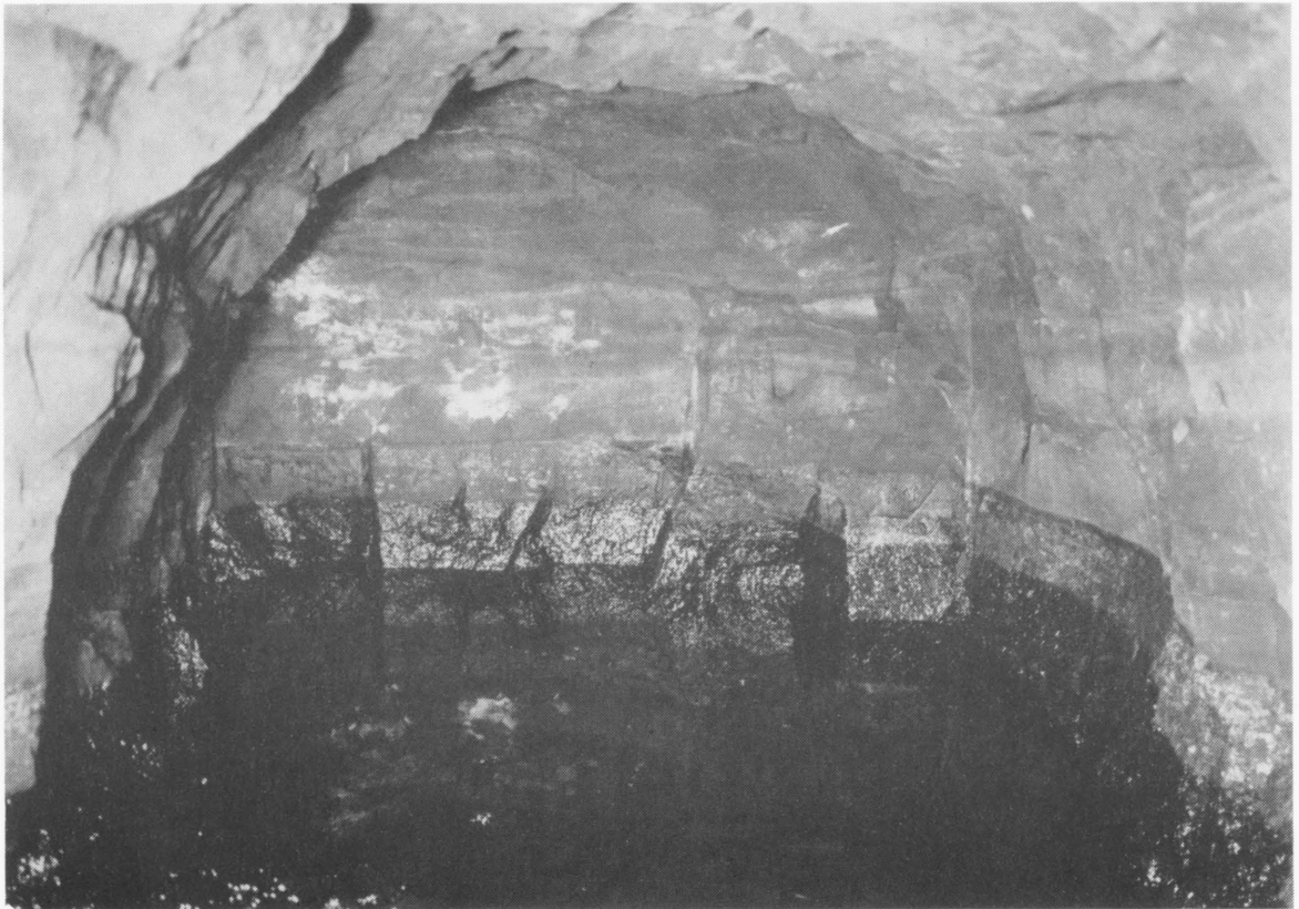
Plate 1b: Coalport Tar Tunnel: natural bitumen draining out of the Thick Rock Sandstone of the Coalport Formation. This pool of tar is 2.4 m square and the back wall of the sump 2.1 m high. (B.G.S.)
